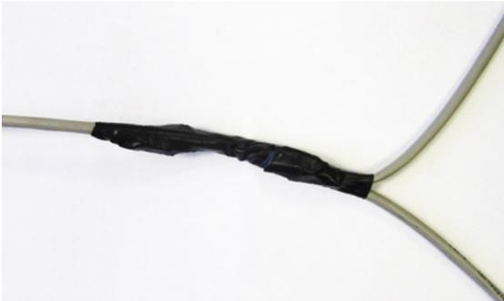
9. Make sure to tape or ziptie all 3 CAT5 lines to the structure to support the 3 way splice and provide strain relief.
